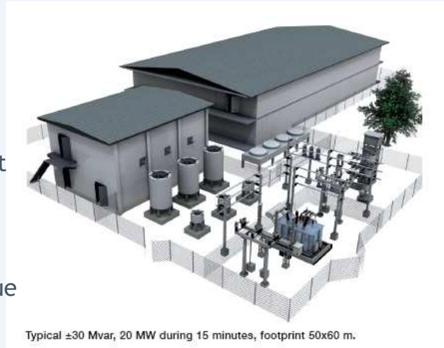
Typical  $\pm 30$  Mvar, 20 MW during 15 minutes, footprint 50x60 m.
