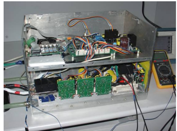
20kVA PM Brushless Inverter
